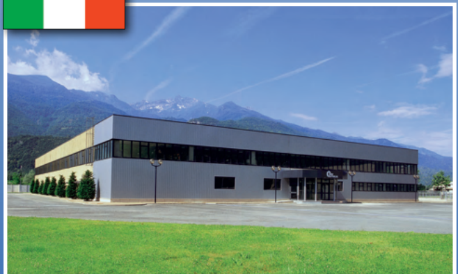
AUTOBLOK manufacturing plant Caprie-Torino
